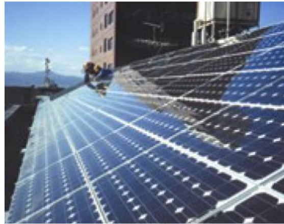
Figure 1. Solar PV Array
